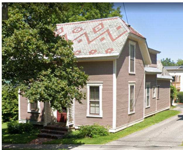
Figure 17. Emma Amanda's house at 274 Maple St, Burlington still standing
